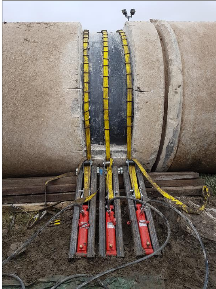
Figure 11. Strain restoration tool installed in Segment B.
